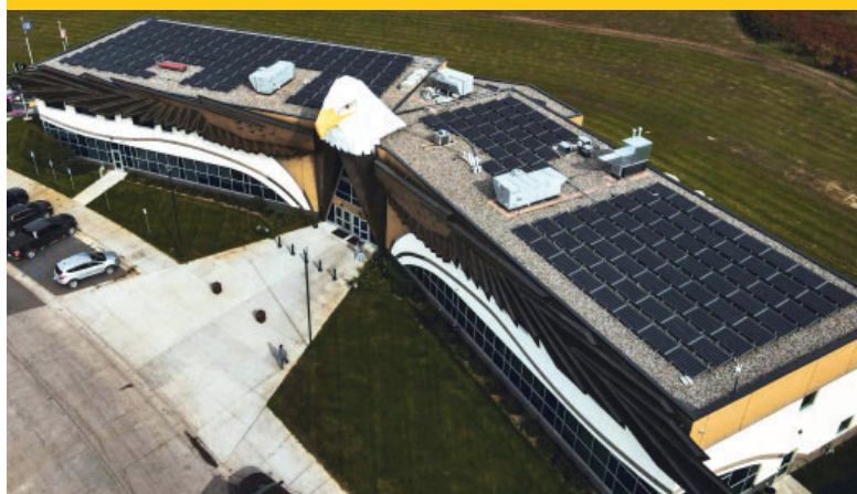
Photo: Red Lake Nation's Government Center, an energy producing & energy storage unit.
